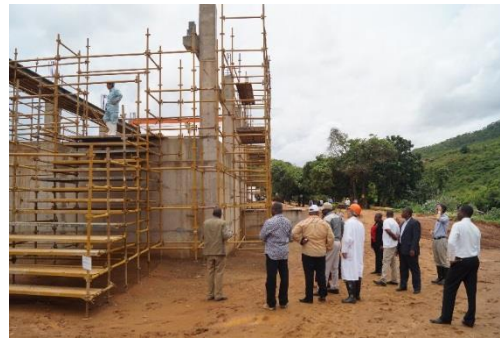
New pumphouse under construction
