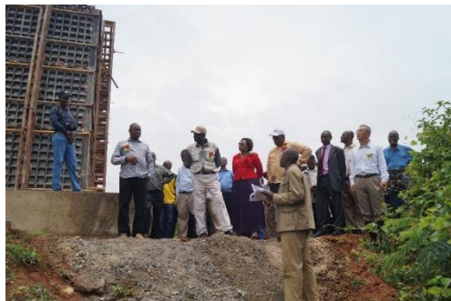
Flood prevention walls being constructed around existing pumphouse
