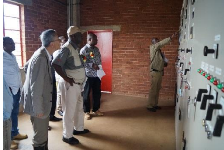
Control room of the pumphouse
