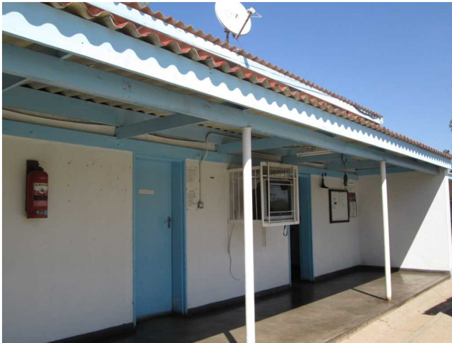
Renovated main ward
