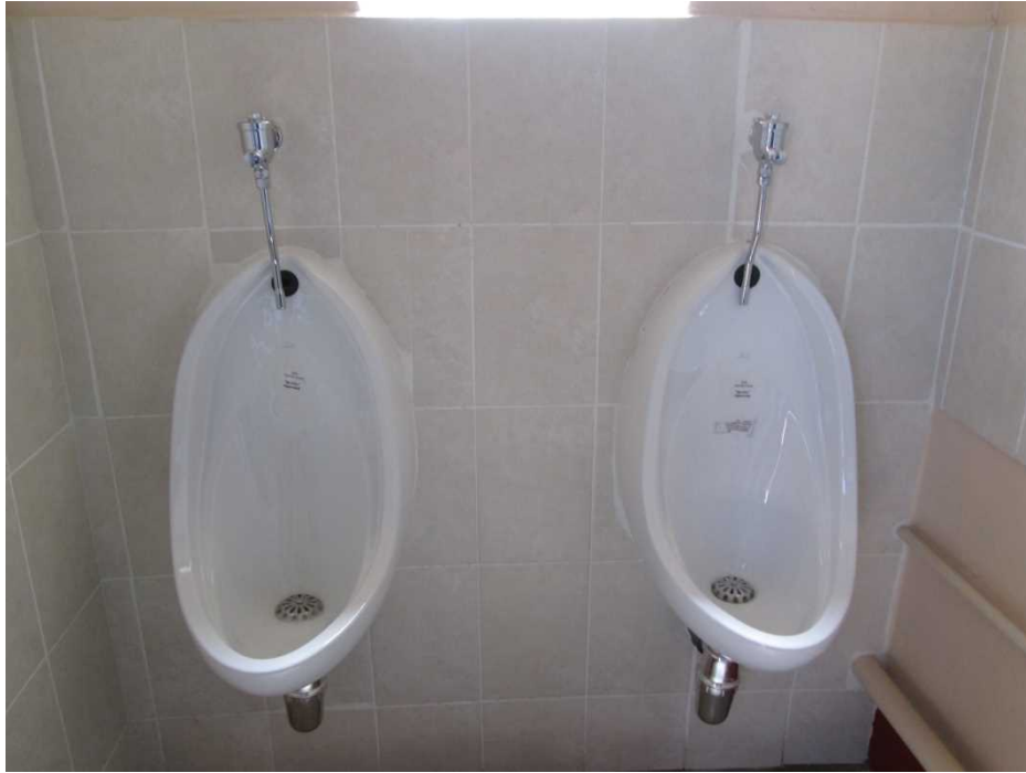
New toilet block
