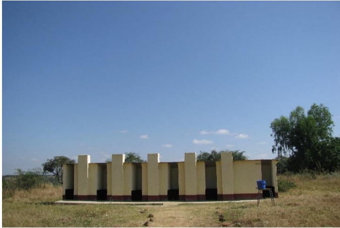
トイレ棟 Completed ablution block
