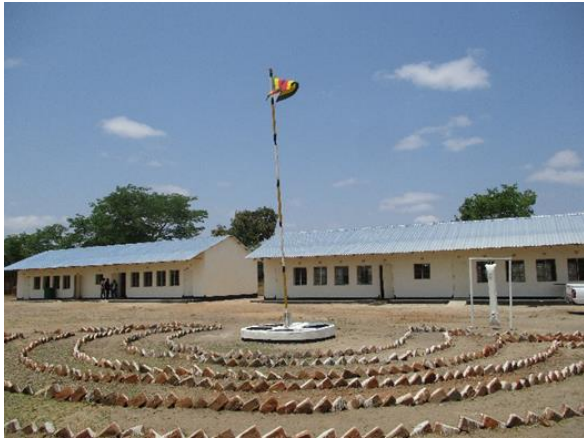
New classroom blocks
