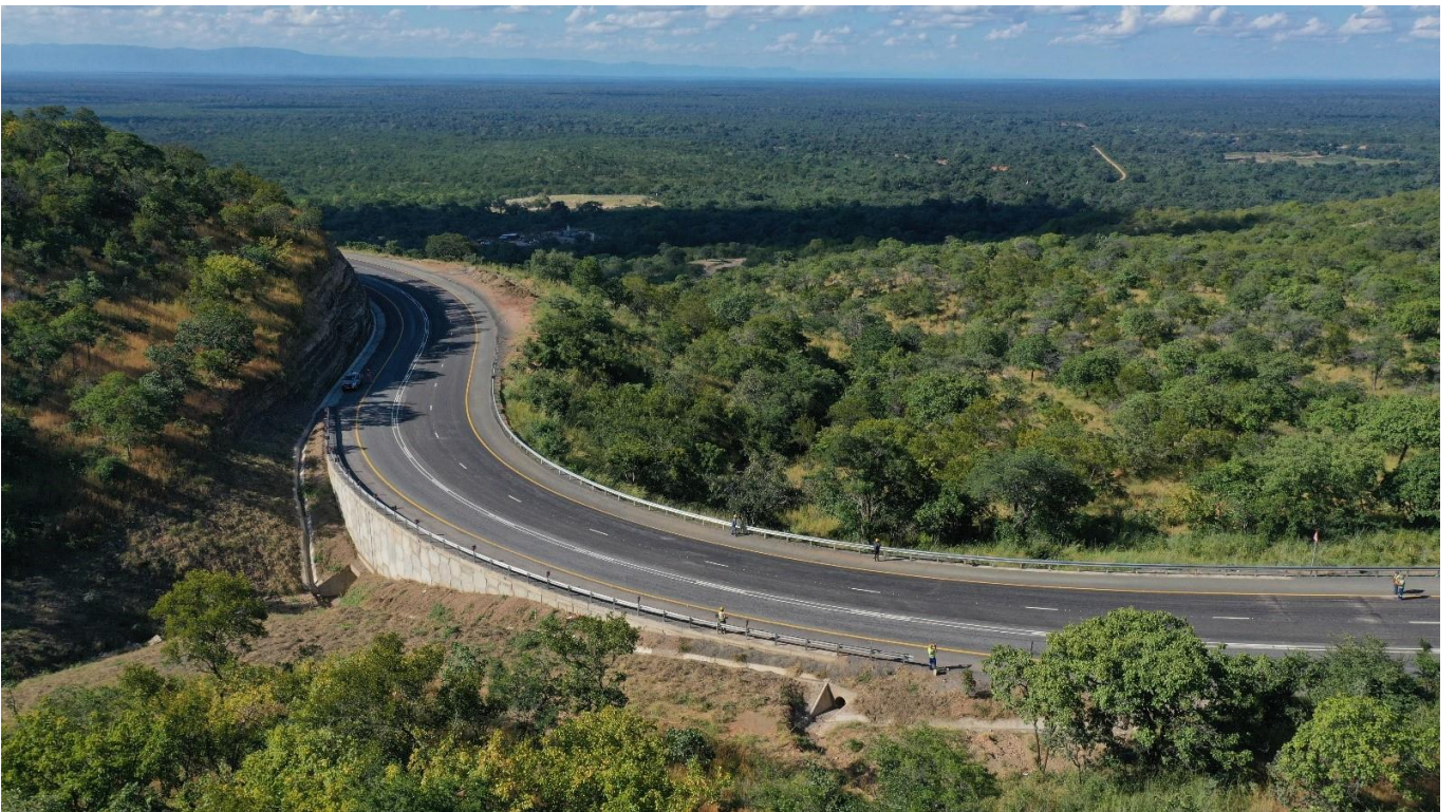
Part of the completed new road section
