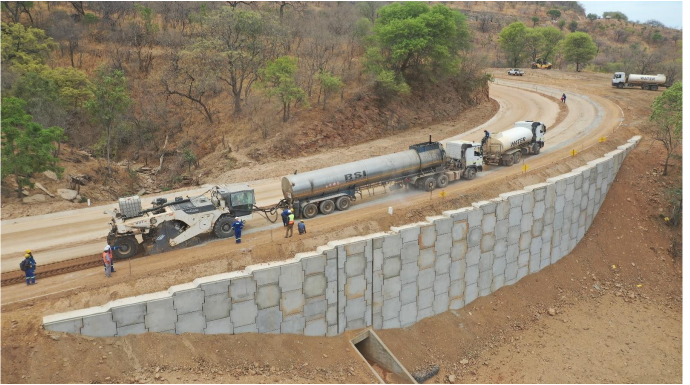
Construction of the improved road section
