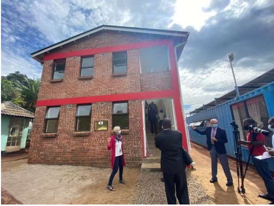
Newly-built Multipurpose Skill Training Centre.
