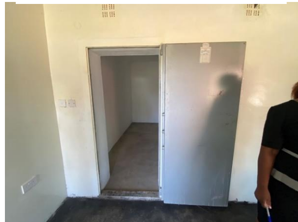
Safe room in a classroom block
