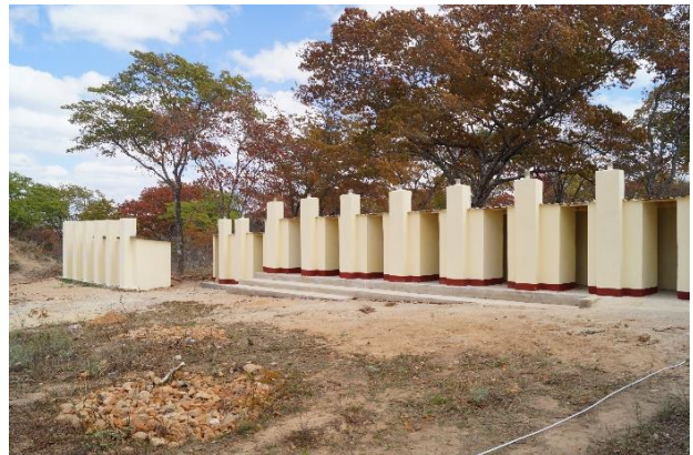
One of the new toilet blocks
