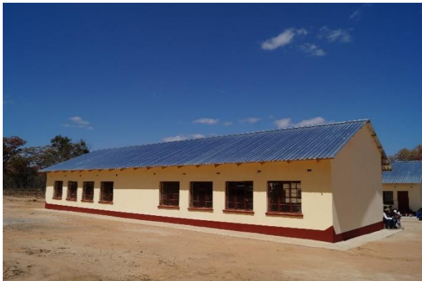
One of the new classroom blocks
